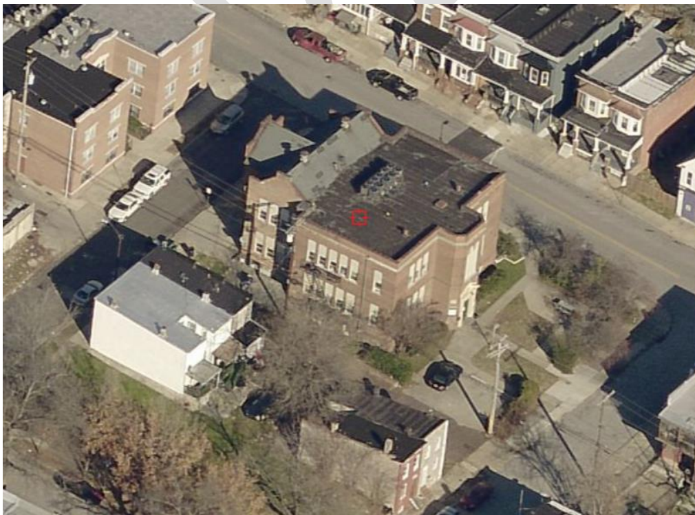
Image 2: 2020 Aerial Photo of property, view from South. (Eagleview)
