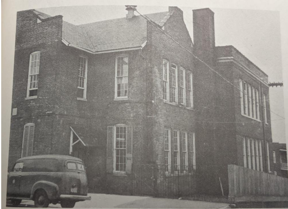
Rear and southwest side of building.
