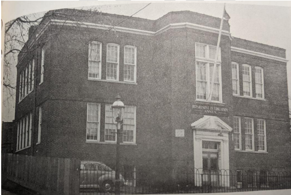
Building faces Kennedy Avenue.
